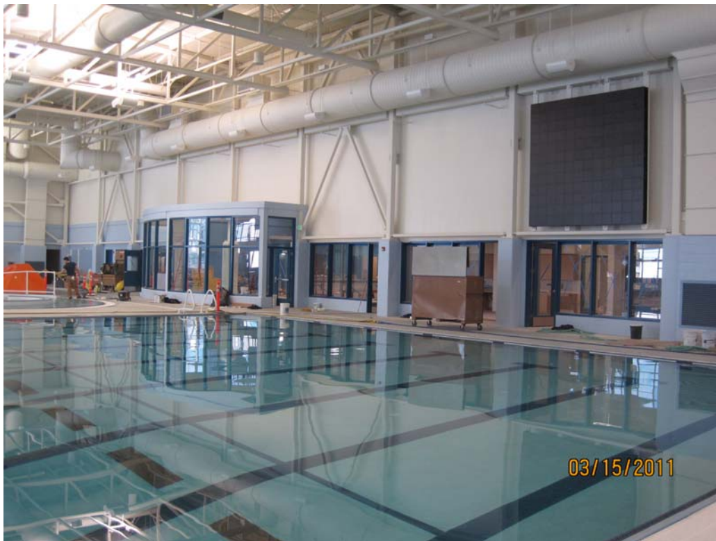
Lap Pool – View Toward Lobby Glass Viewing Area and Private Rooms
