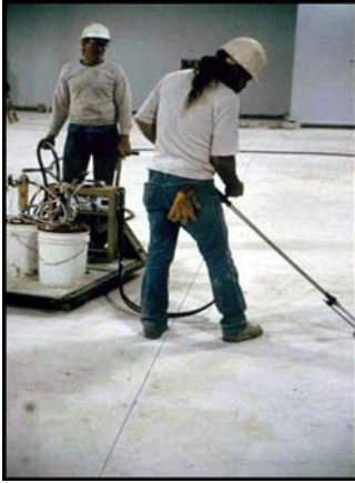
Figure 12: Joint filling
