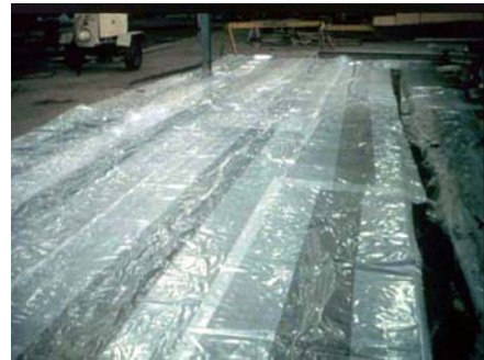
Figure11: Wet cure with poly sheet
