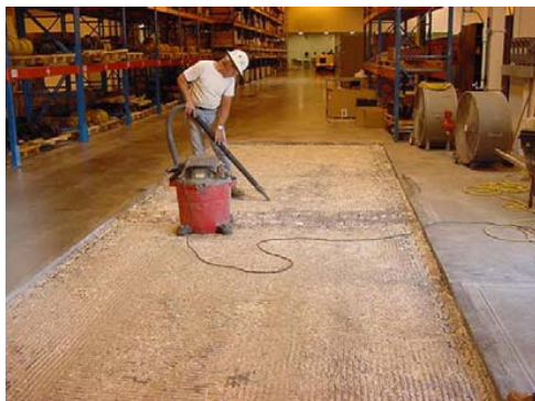
Figure 3: Preparing existing slab
