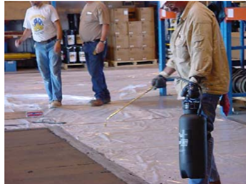
Figure 1: Applying Confilm ®
