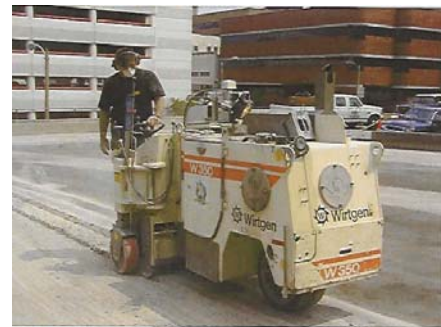
Figure 4 Milling existing concrete surface
