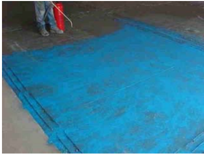
Figure 8 apply Liquid Surface Etchant ®
