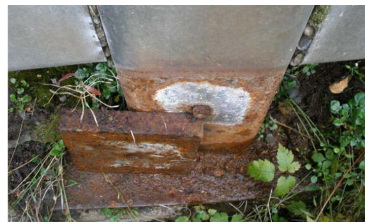
16 TIE ROD REPAIR PER DETAIL 4/S101, STA. 16+01 LEFT
