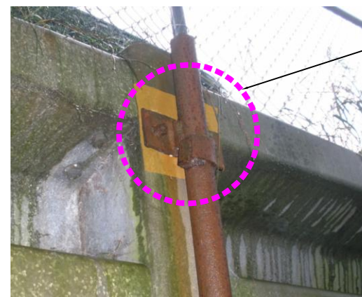
13 TYPICAL RUSTED PIPE AND BRACKET
