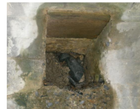
17 12" SQUARE OPENING - TO BE PLUGGED WITH CONCRETE
