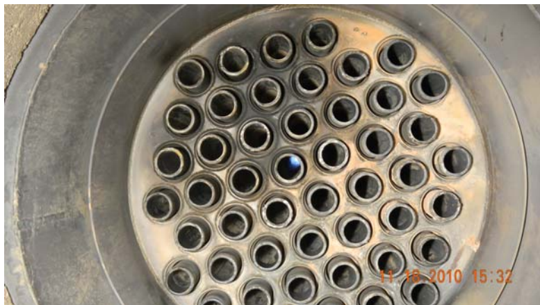
Photo 2: Looking up at lower end tube repair area
