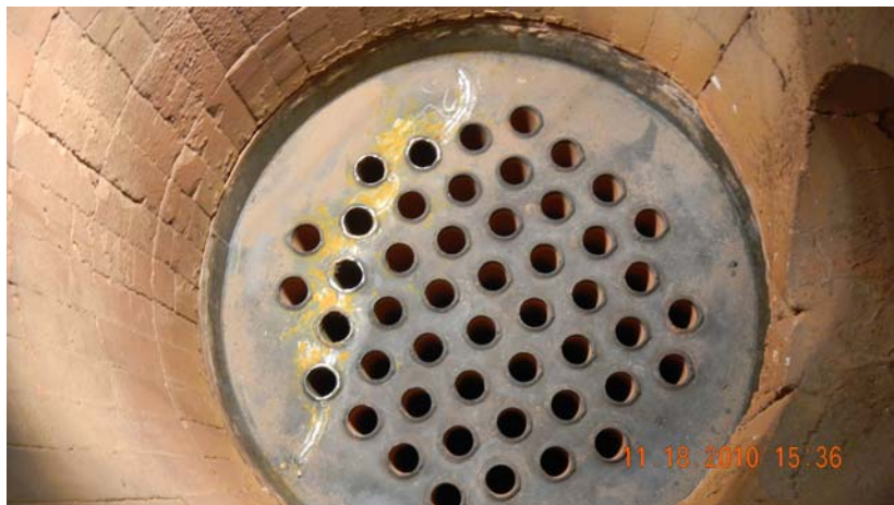
Photo 5: Upper end tube repair area as seen from above
