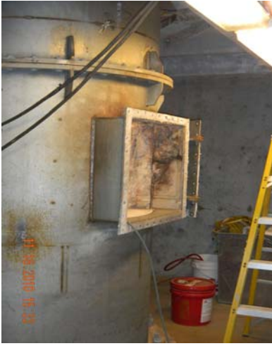
Photo 1: Access to lower end tube repair area
