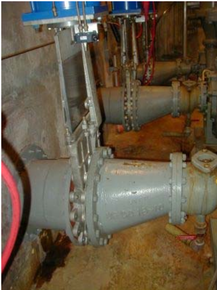
Outer Drive – Pump Suction Pipes
