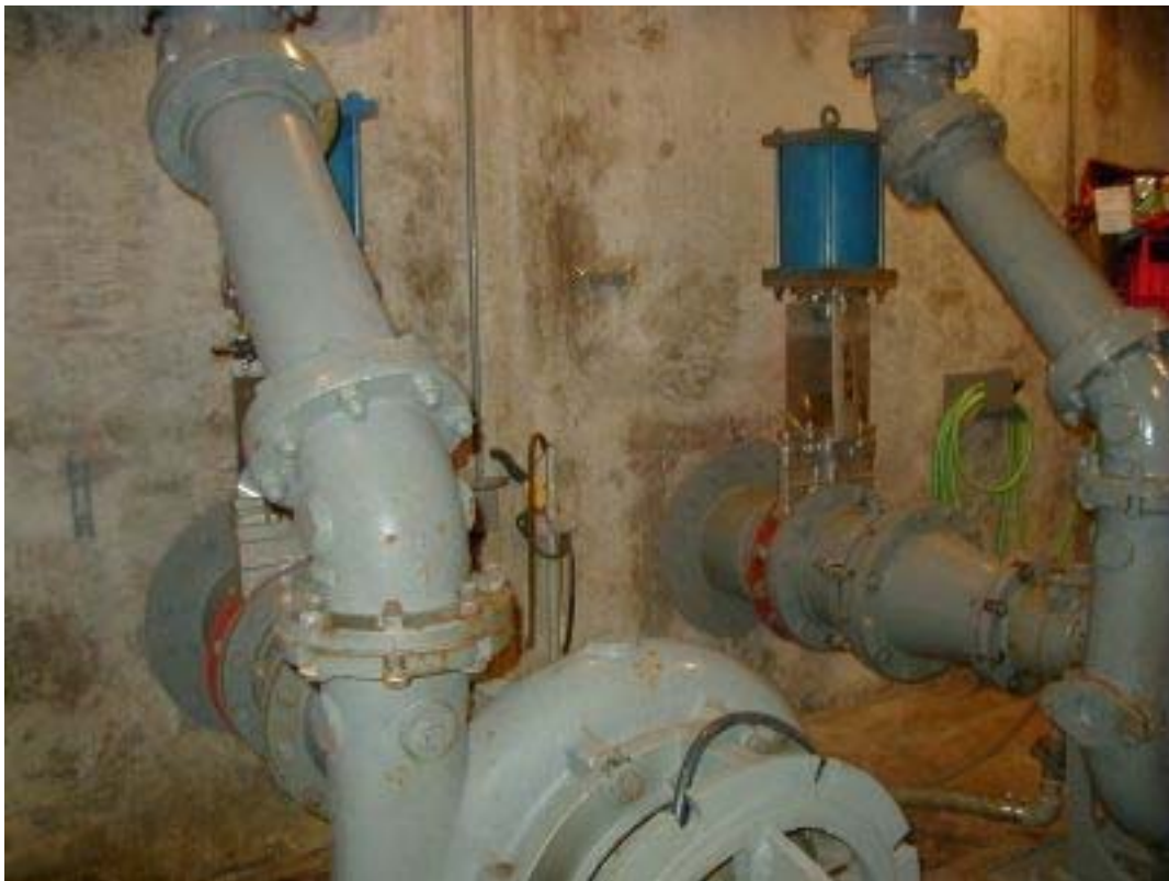
West Juneau – Pump Suction Pipes
