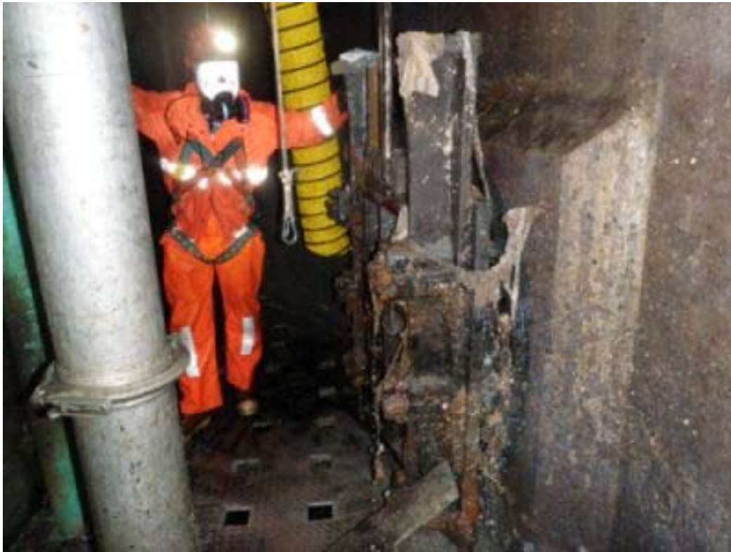
Outer Drive - Influent Slide Gate Installation
