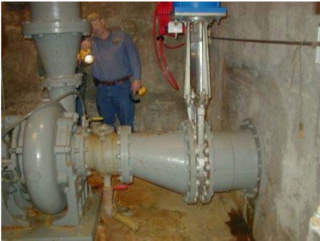
Outer Drive – Pump Suction Pipe
