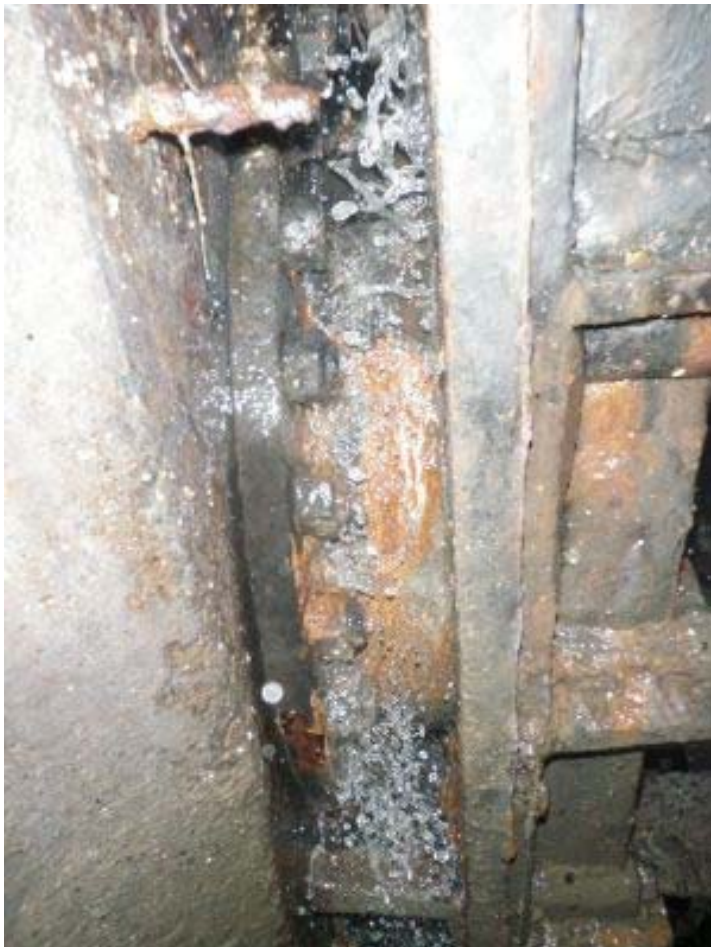
Outer Drive – Influent Slide Gate, Pipe Flange
