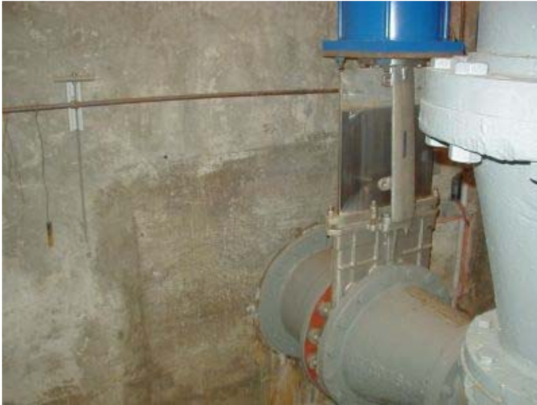
Outer Drive – Pump Suction Pipe Wet Well Penetration
