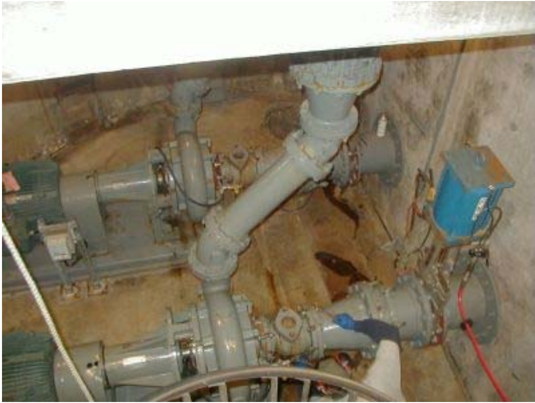
West Juneau – Pumps and Suction Pipes
