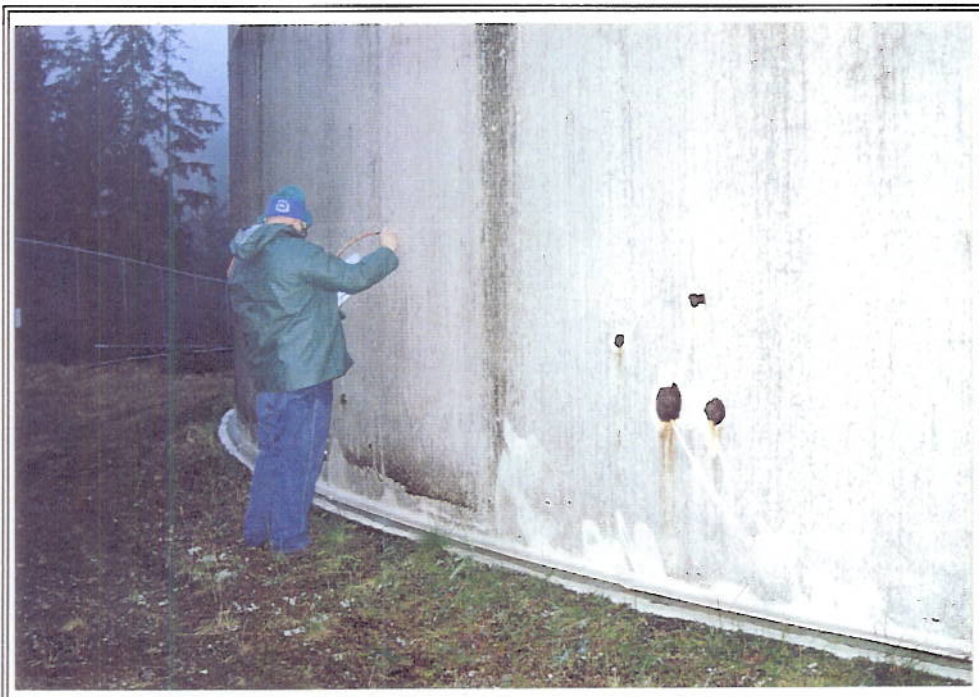
PHOTO No. 2: Tier C, Ground Panel, 7:30 Position - Note the four areas of coating failures with corrosion and the otherwise good condition of the protective coating. The inspector is taking ultrasonic thickness measurements of the steel.
