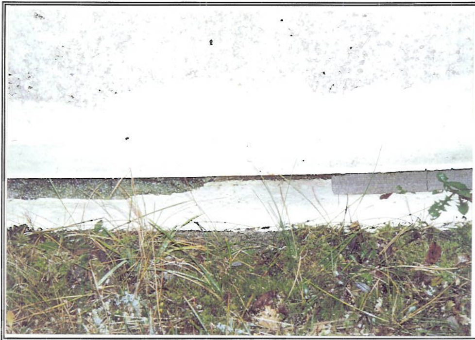
PHOTO No. 5: Ringwall Foundation, 2:00 Position - Note the small section of the grout that is missing from between the bottom flange of the tank and the concrete ring foundation. This condition was found to be typical around the perimeter of the tank.
