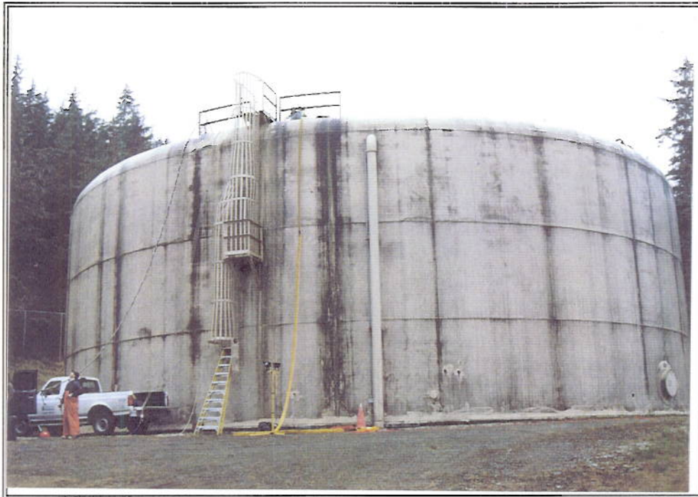
PHOTO No. 1: Auke Lake Tank, General View - Note the arrangement of the ladder, overflow pipe, and access man hole. The dark streaks apparent on the tank are dirt in areas of runoff. The tank coating was found to be greater than 99% intact.
