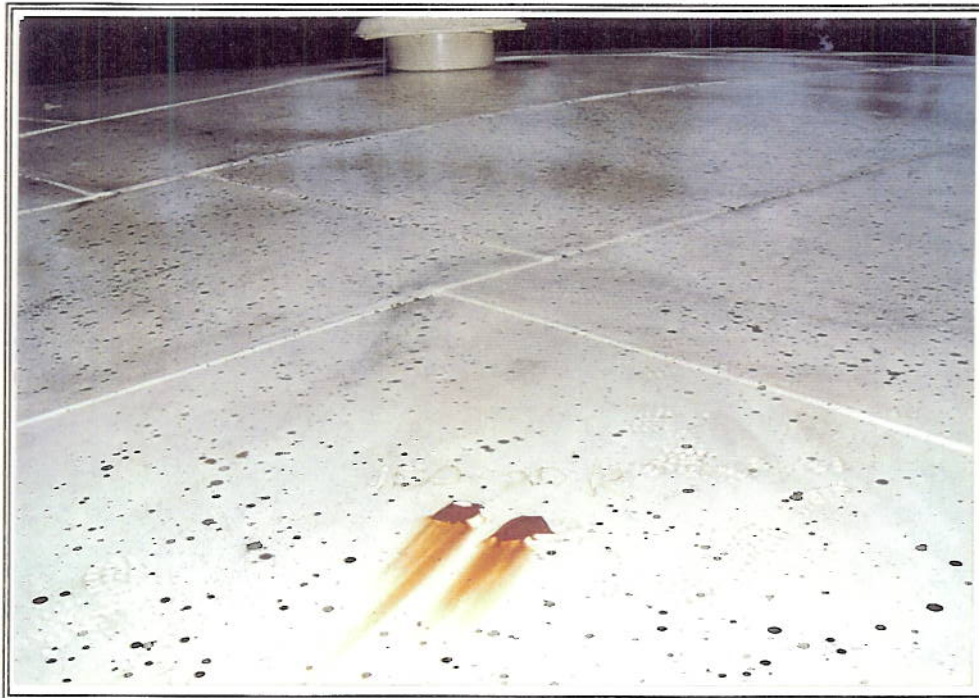
PHOTO No. 3: Tank Top, 1:30 Position - Note the two areas of coating failure with corrosion. Measurement showed both areas to be less than 6 inch in diameter. Note the center roof vent in the distance (top center).
