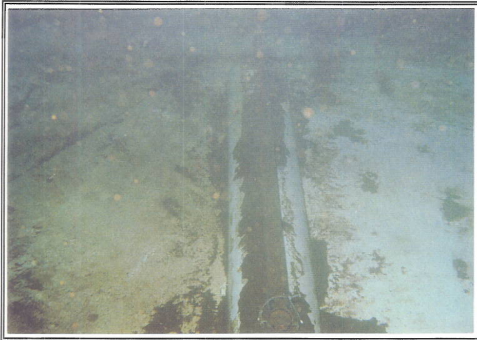
PHOTO No. 9: Tank Interior, Bottom - Note one of the cathodic protection system anode attached to the bottom. The anode is supported atop a semi-cylindrical PVC base. Inspection did not reveal any damage to the anodes.
