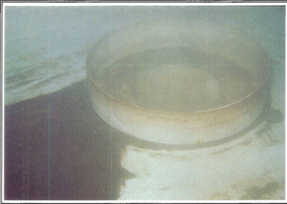
PHOTO No. 6: Tank Interior, Bottom, Tank Outlet - Note the good condition of the coating on the tank outlet and the floor of the tank. Sediment, typical of that removed from the tank can be seen to the left of the outlet pipe. Additional cleaning and sediment removal was conducted prior to inspection of the tank floor.
