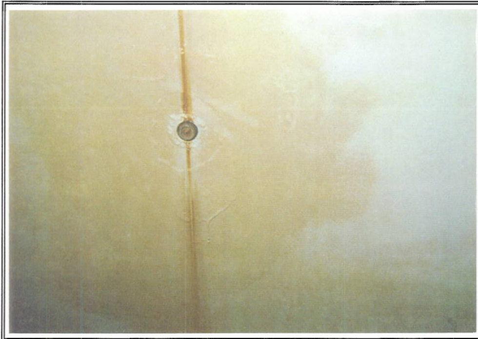
PHOTO No. 10: Tank Interior, Tier C, Bottom Panel, 11:50 Position - Inspection showed the cathodic protection system reference cell to have been broken off flush with the tank wall.
