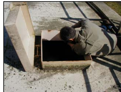
11 Access hatch in front of ladder
