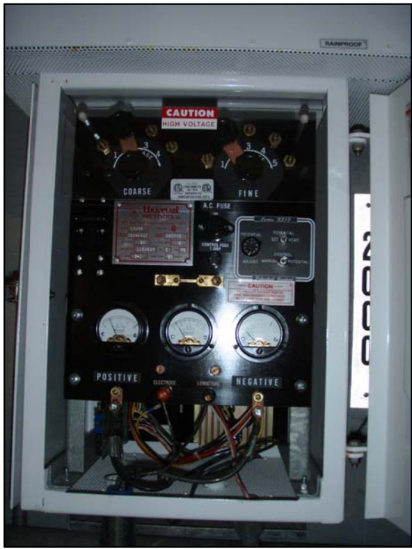
11 Inside cathodic rectifier, photo 7, above.
