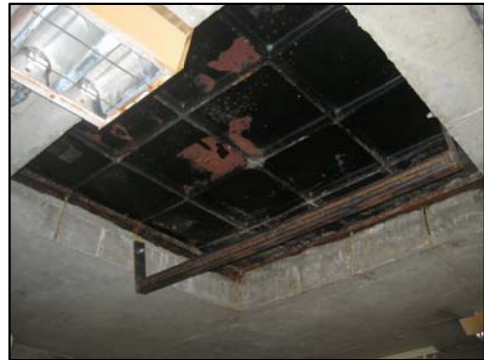
5 Underside of steel equip. cover
