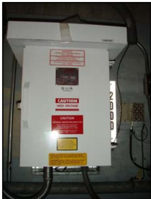
7 Cathodic protection panel on wall
