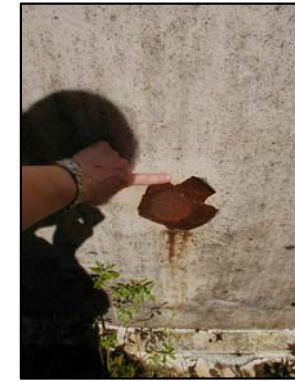
10 Surface corrosion-approx dia. 6"
