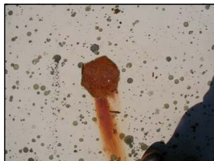
13 Sample of 6" dia. corrosion spot
