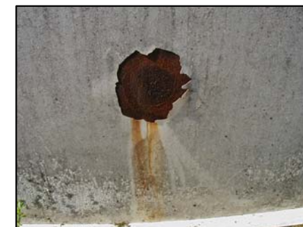
16 Sample 6" diameter corrosion spot
