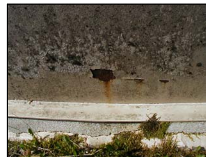
15 Sample corrosionat grout ring
