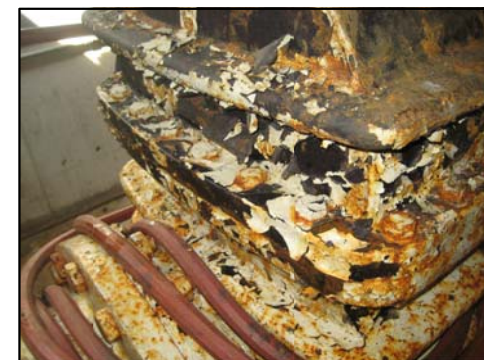
8 Paint on valve box down to blackiron
