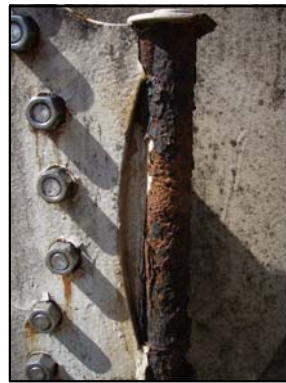
2 Hinge at 24" side access manhole
