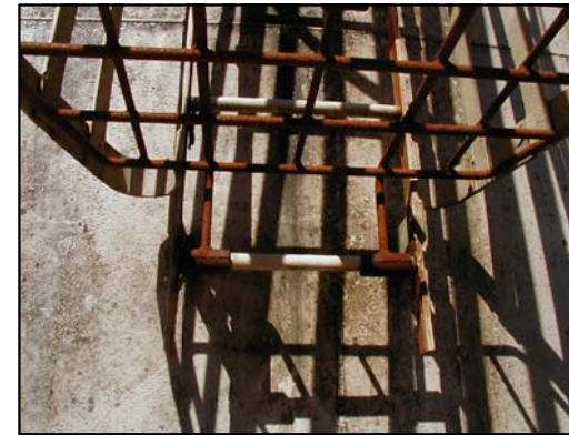
8 Corrosion at access ladder
