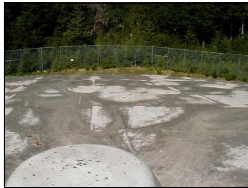
6 Sample corrosion on top of tank
