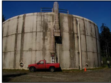
1 Access ladder, overflow pipe & side access manhole
