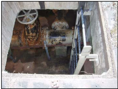
2 View into valve vault
