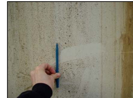
12 Algae cleaned on side of tank
