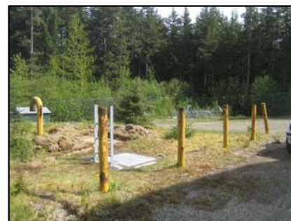
15 Vent and five pipe bollards
