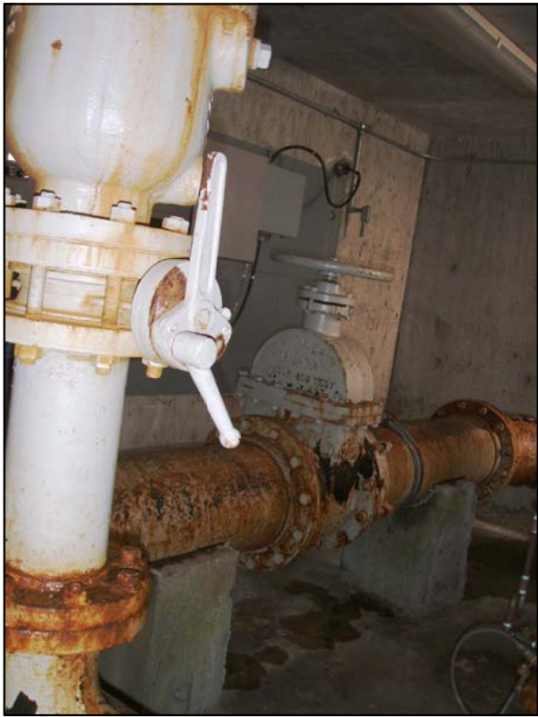
10 Note condensation on exist. pipe
