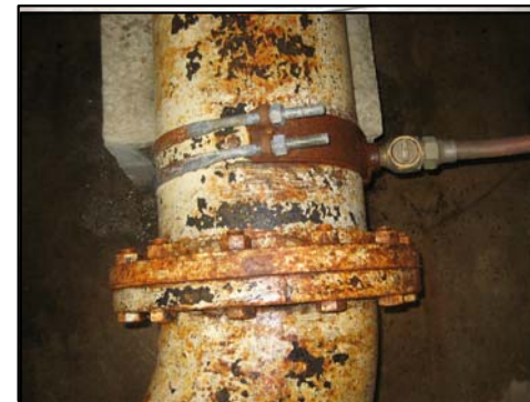
12 Pipe with grounding strap
