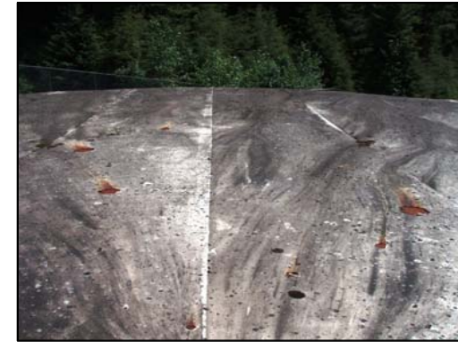
4 Corrosion spots - 6" average diameter
