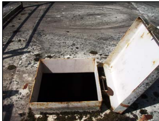
7 24" square tank access hatch
