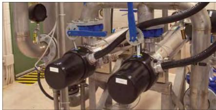
Developed using advanced Computational Fluid Dynamic (CFD) modeling, and incorporating high-output amalgam lamps, the TrojanUVSwift™SC is extremely space efficient. Its compact footprint allows the system to be integrated into restrictive pipe galleries of water treatment facilities – vertically or horizontally – reducing installation costs and eliminating the need for additions to buildings.
