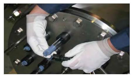
The TrojanUVSwift™SC design simplifies maintenance procedures. For example, lamp changeovers require no tools and take less than five minutes per lamp.
