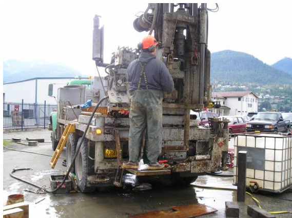
Different drilling techniques employed to drilled to the granular layer. Solid auger was used to drill through A-J fill, while bentonite mud was used to help stabilized the boreholes. Casing were also added at full borehole lengths to prevent caving-in.
