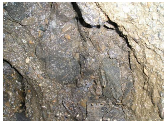
Figure-4. The thick A-J rockfill layer. Shot taken at the side of the collapsed TH-3.
