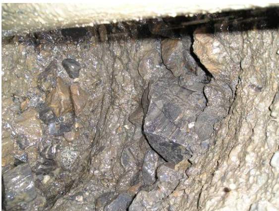
The A-J rockfill layer. In these photos, the voids typically within the rock fill were already filled with drill cuttings and bentonite mud.
