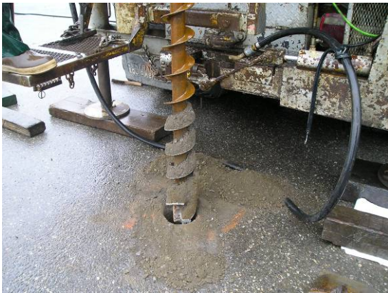
Different drilling techniques employed to drilled to the granular layer. Solid auger was used to drill through A-J fill, while bentonite mud was used to help stabilized the boreholes. Casing were also added at full borehole lengths to prevent caving-in.
