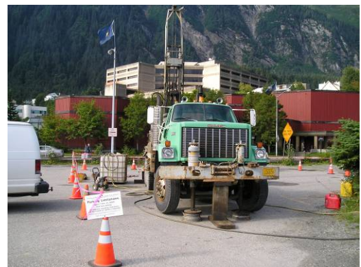
Figure-3. R&M's CME-55 truck-mounted drill rig working in TH-4.
