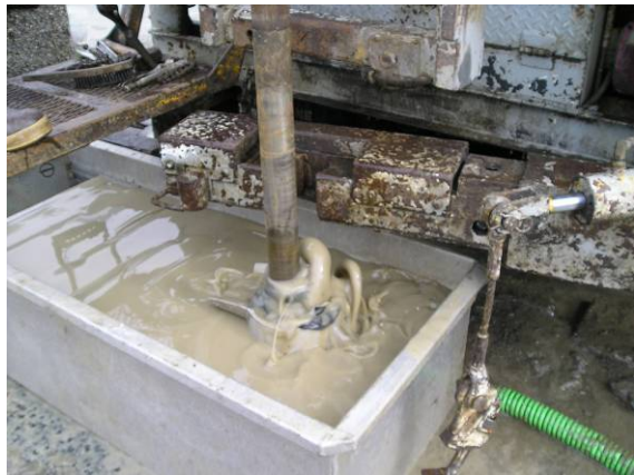
Different drilling techniques employed to drilled to the granular layer. Solid auger was used to drill through A-J fill, while bentonite mud was used to help stabilized the boreholes. Casing were also added at full borehole lengths to prevent caving-in.
