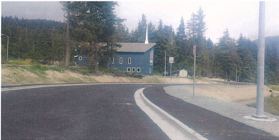
View North along Karl Reishus Boulevard toward subject subdivision
