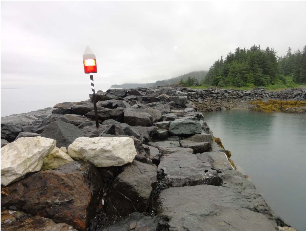
PHOTO 7 – LOOKING NORTH FROM END OF SUBJECT BREAKWATER. (071317_0874)
