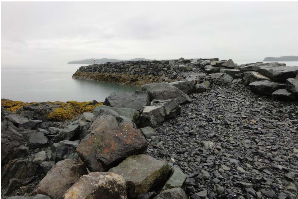
PHOTO 6 – LOOKING SOUTHERLY FROM UPLANDS TOWARDS SUBJECT BREAKWATER SITE SHOWING EAST SIDE OF BREAKWATER. (071317_0870)
