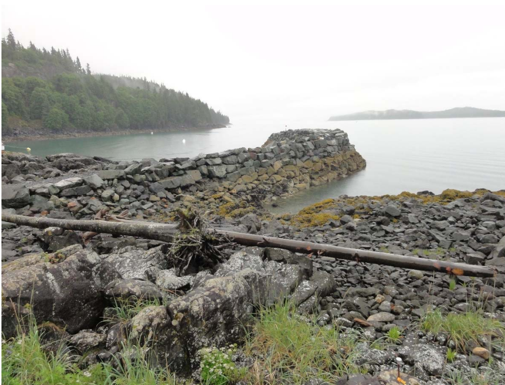
PHOTO 8 – LOOKING SOUTH AT WESTERLY SIDE OF BREAKWATER. (071317_0877)
