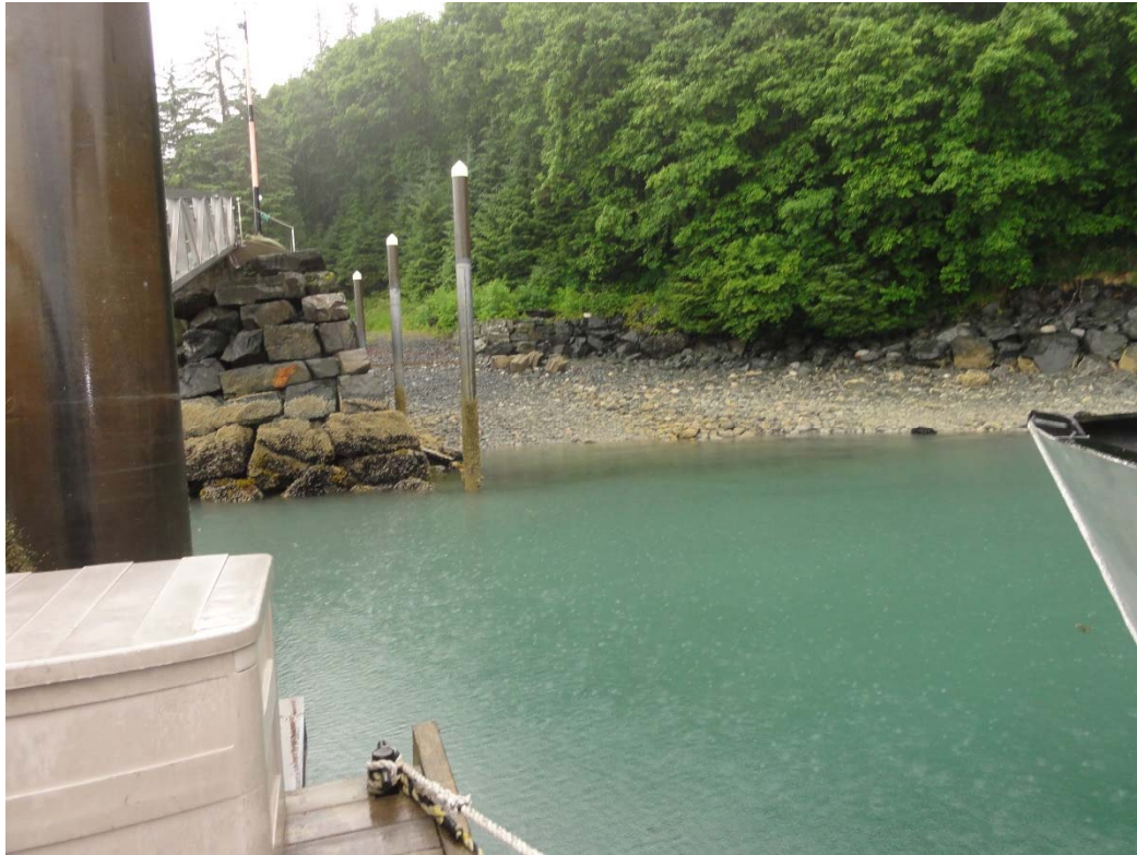
PHOTO 4 – LOOKING NORTHERLY ALONG SUBJECT SUBMERGED LANDS AND ADJACENT UPLANDS AT GRAVEL RAMP ALONG EASTERLY SIDE OF DOCK SITE. (071317_0857)
