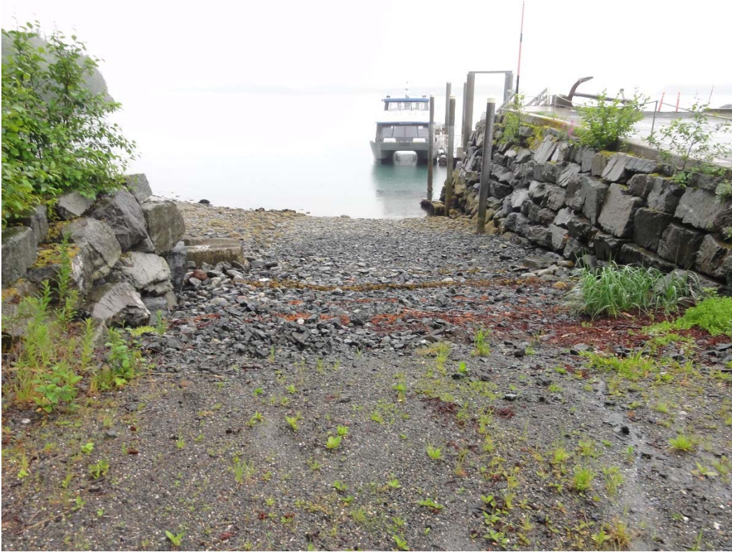
PHOTO 5 – LOOKING IN THE OPPOSITE, SOUTHERLY DIRECTION DOWN SLOPING RAMP AT EASTERLY SIDE OF DOCK SITE. (071317_0859)
