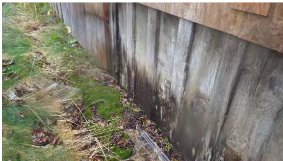
Moisture damage under windows
