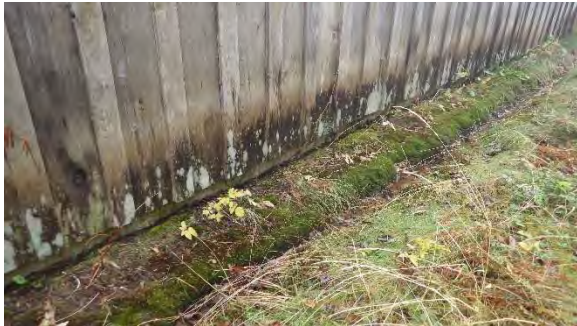
Moisture damage at base of exterior siding south section
