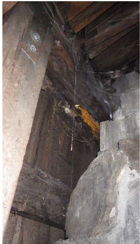
Deteriorated wall framing behind chimney
