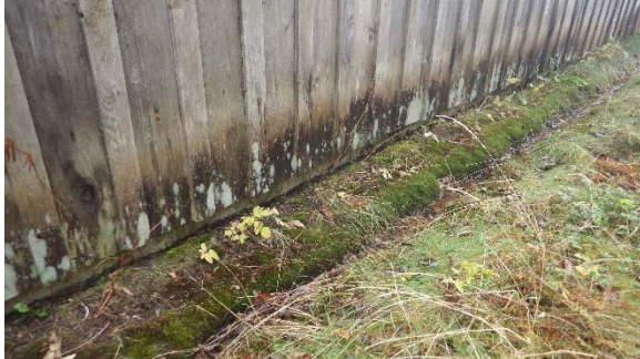
Moisture damage at base of exterior siding south section
