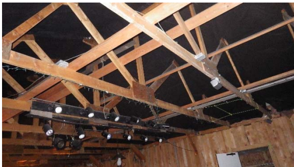
Middle section roof trusses
