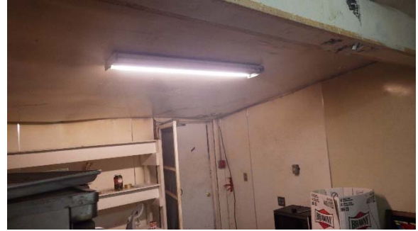
Uneven ceiling in kitchen area- gypsum wall board attachment is failing.
