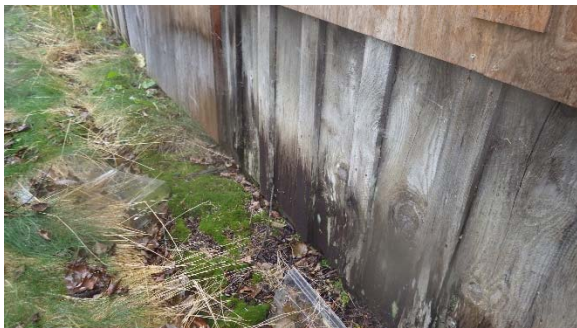
Moisture damage under windows
