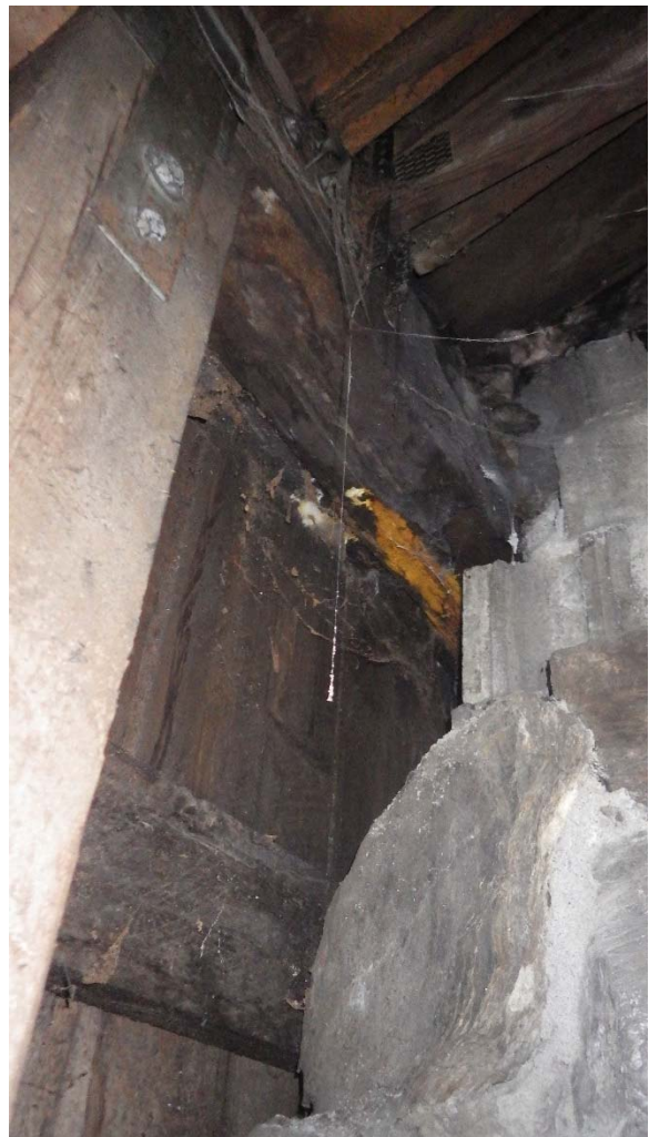
Deteriorated wall framing behind chimney
