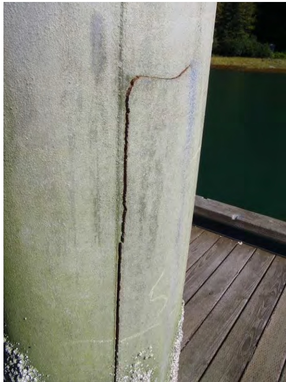
Split pile M6 on main float.
