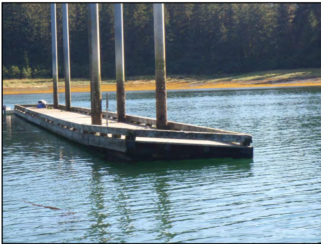
Raised corner of Stockade Point float.
