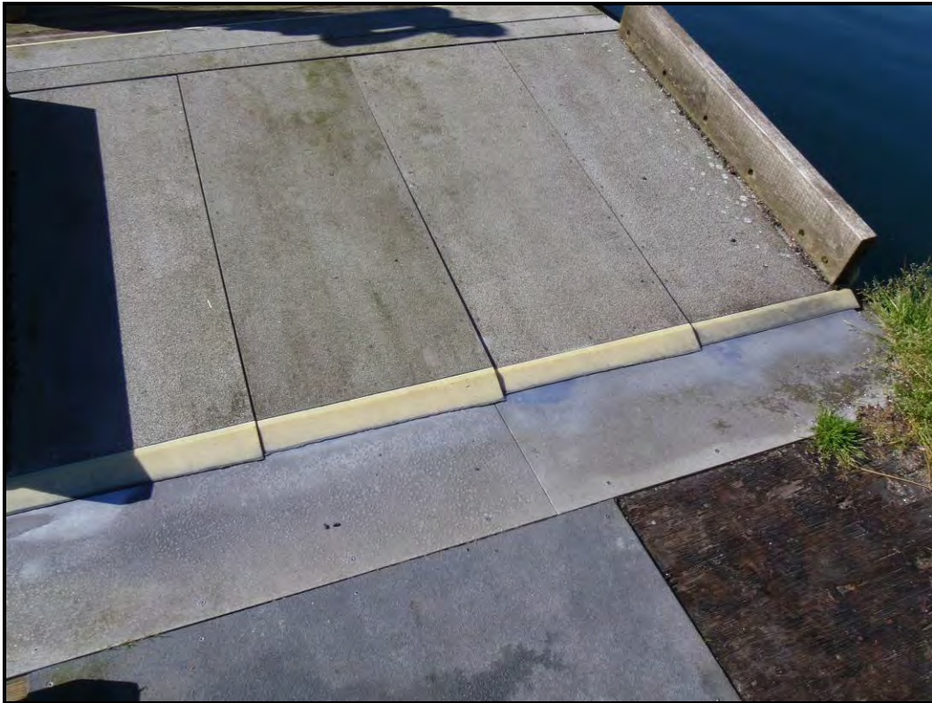
Transition plate assembly – worn UHMW nosing pieces.
