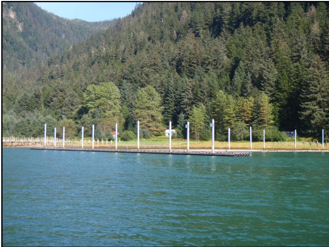
Overall view (face of main float) of mooring pile height differential due to ice jacking.
