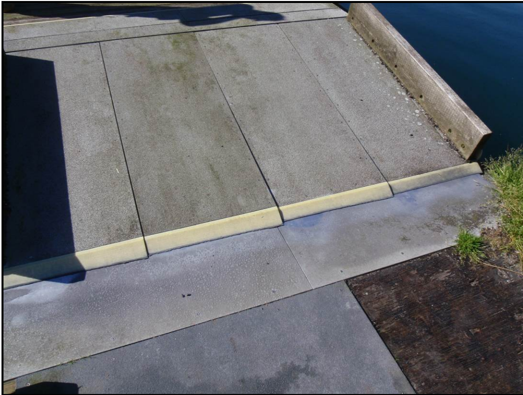
Transition plate assembly – worn UHMW nosing pieces.
