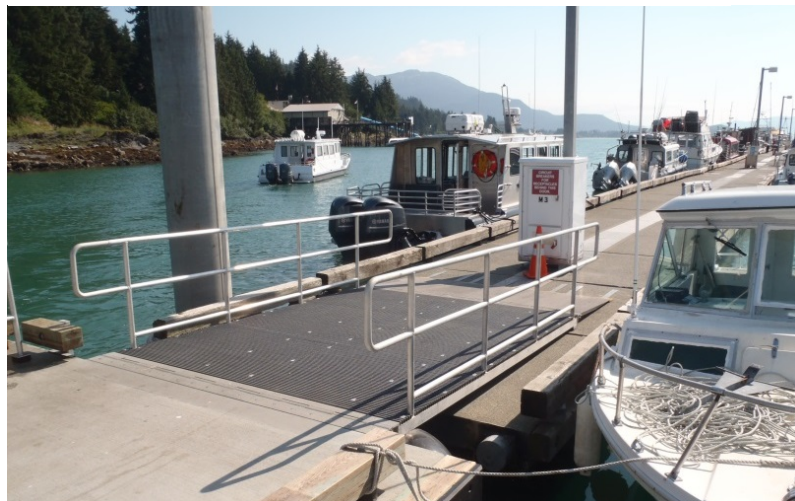
FIGURE 2 TRANSITION RAMP - 2 TO EXISTING CONCRETE DOCK
