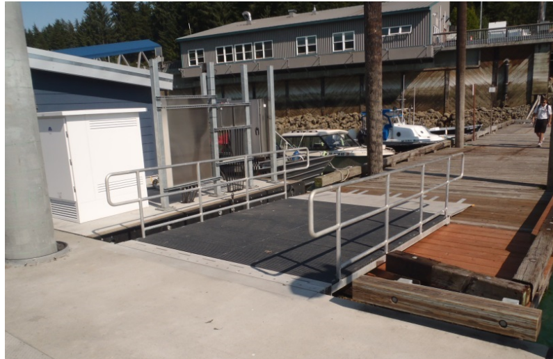
FIGURE 1 TRANSITION RAMP - 1 TO OLDER WOOD DOCK
