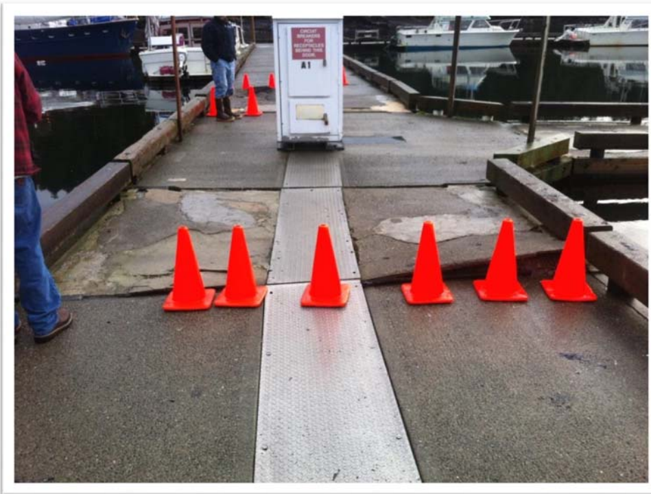
Figure 2: Crushed Float Module #2
