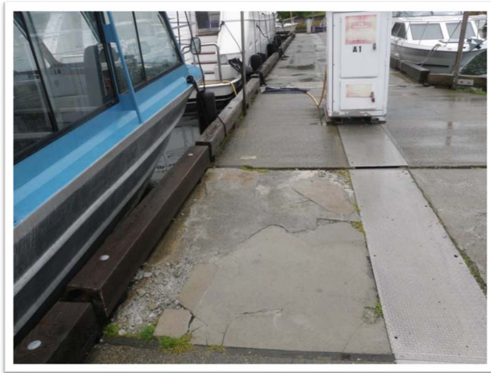
Figure 3: Previous Damage to Float Deck Prior to Failure (Photo taken in 2011)
