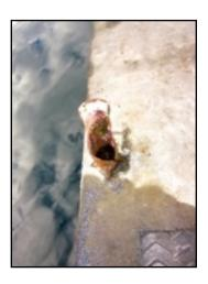
8. Found: All hatches are missing bolts, in need of gasket maintenance, cleanup and re-coating with painting.
