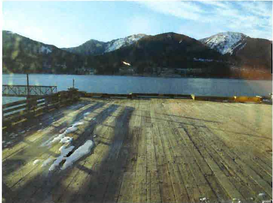
Facing westerly viewing Douglas cruise ship berth and associated dock.
