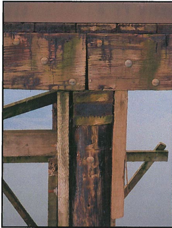
Supplemental stringer bearing detail.
