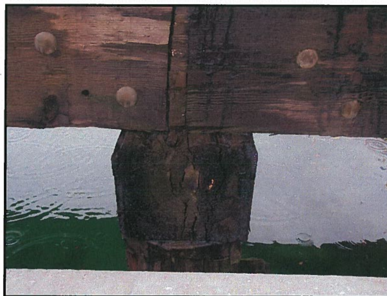
Minimal bearing of stringer on degraded pile cap.
