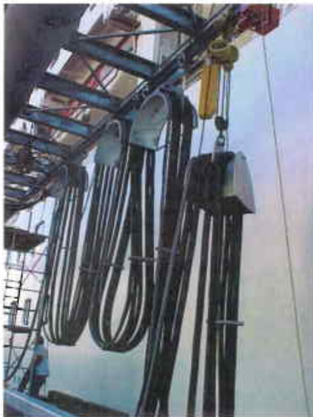
Figure 3 - Shore tie Cable Festoon
