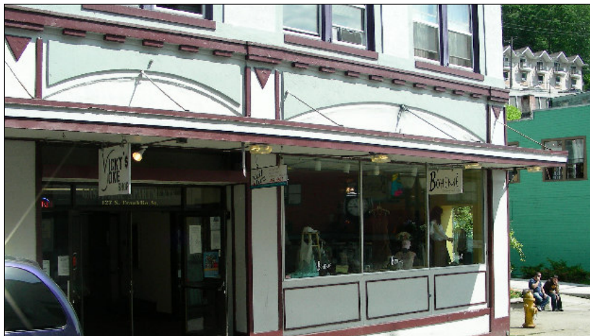
The transoms on the building above have been covered. Although they reflect the openings that were once located there, a more appropriate treatment would be to reopen transoms. Compare with photos on page 15 and 17.
