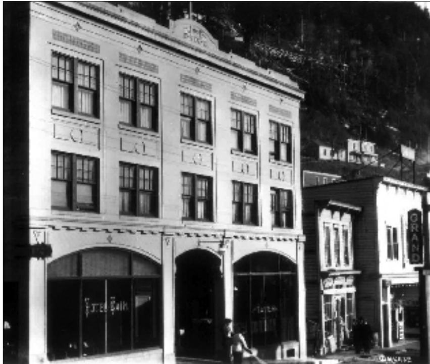
The Hotel Cain (1913, 127 S. Franklin Street) was constructed with reinforced concrete and is an example of the Early 20th Century Commercial Style.
