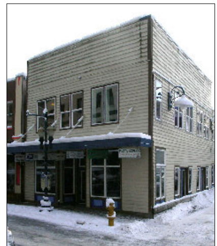
Protect wood siding and other wood surfaces with a painted finish.
