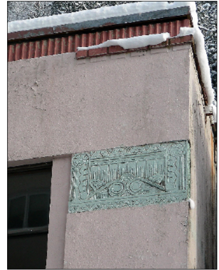
A decorative panel serves as a cap to a vertical attached column, or pilaster, a typical Art Deco detail.
