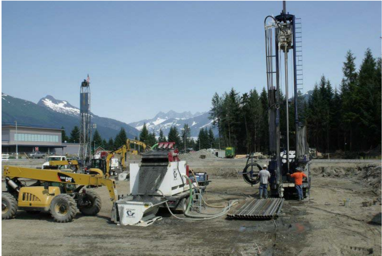
Drilling to establish the vertical ground loops at the Juneau Valley Dimond Park Aquatic Center
