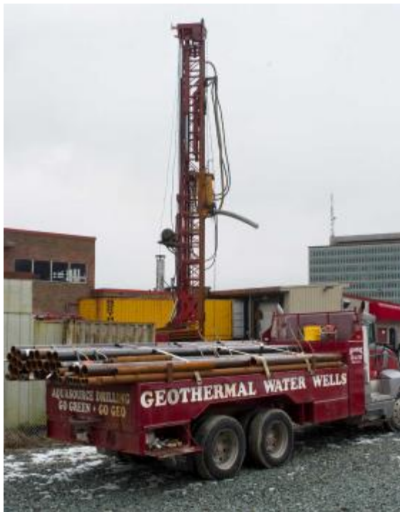
Michael Penn/Juneau Empire Drilling for the new Alaska State Library, Archives and Museum building's geothermal heating system
