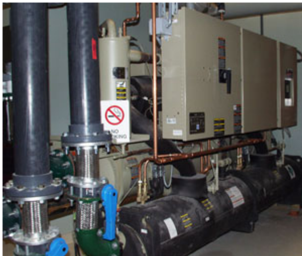
Photo Credit: NOAA - One of two heat pumps that extract 4 degrees of heat from 38-degree seawater and use that energy to heat the 66,000-square foot Ted Stevens Marine Research Institute in Juneau, Alaska.
