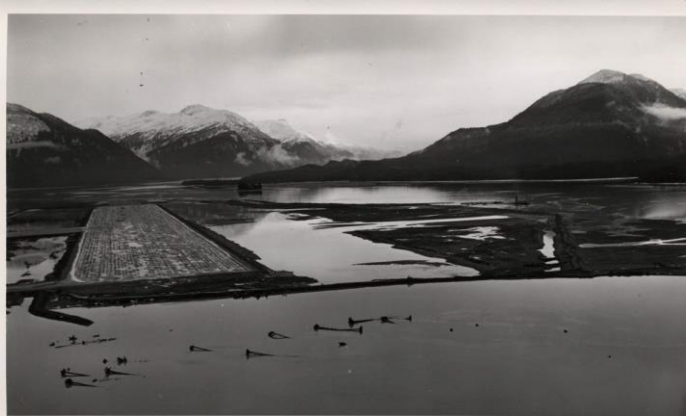
1939 Civil Conservation Corps clearing stumps and debris on flats to extend airfield
