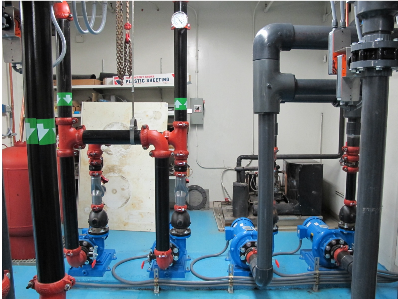
High-Efficiency Circulation Pumps Move Glycol and Water Through the Heat Pumps
