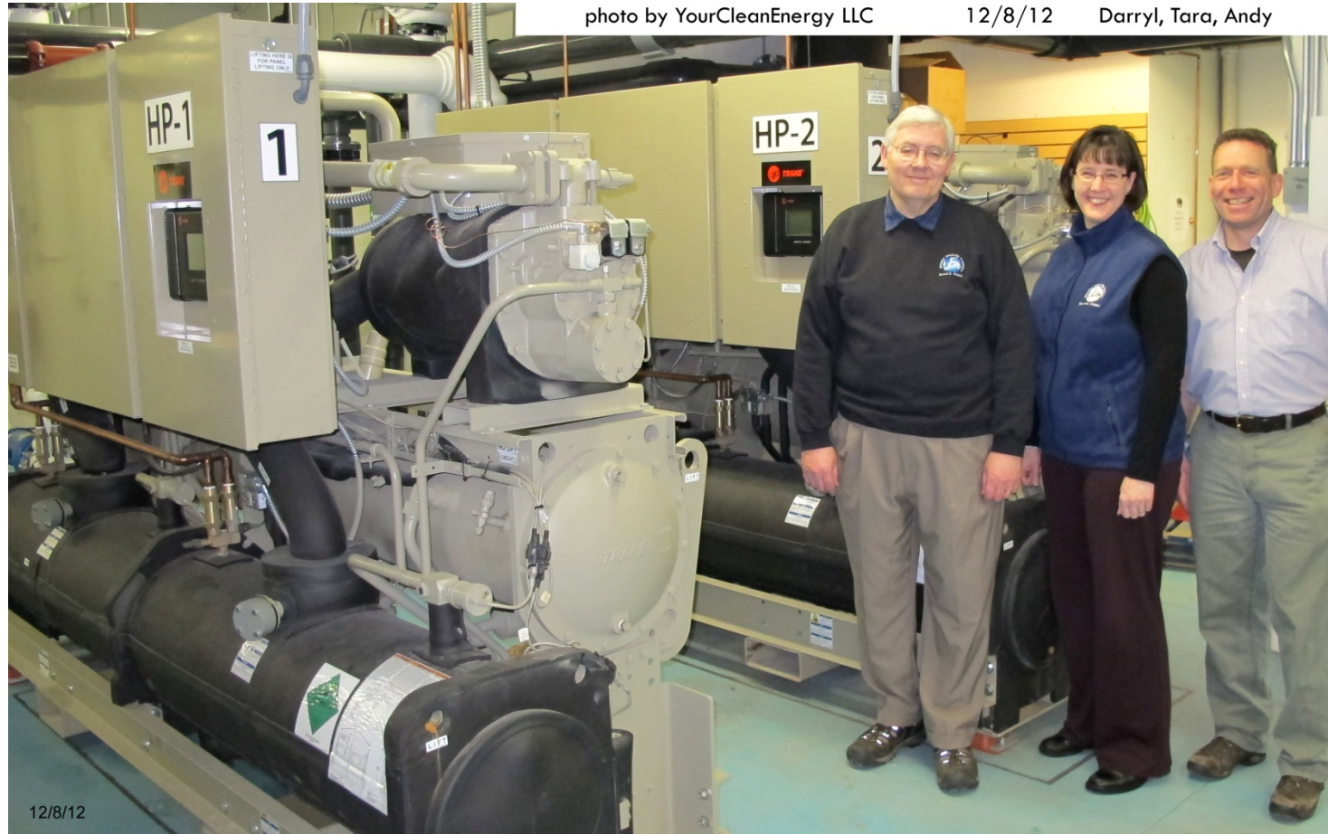
Two 90-Ton Heat Pumps – One or Two Heat Pump Operation
