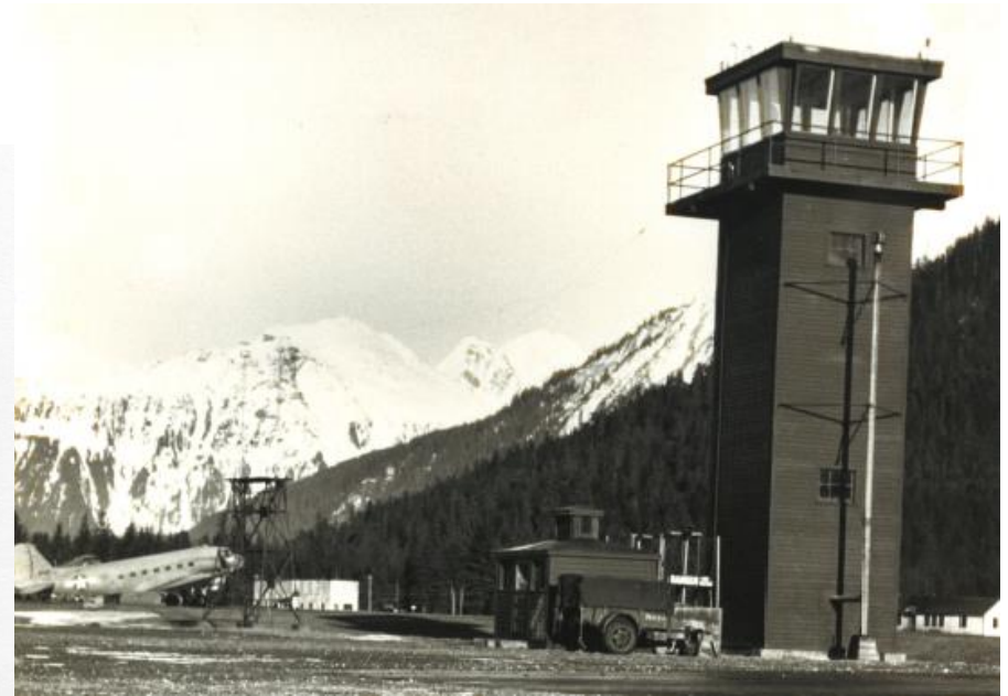
Construction of first Tower by 1943
