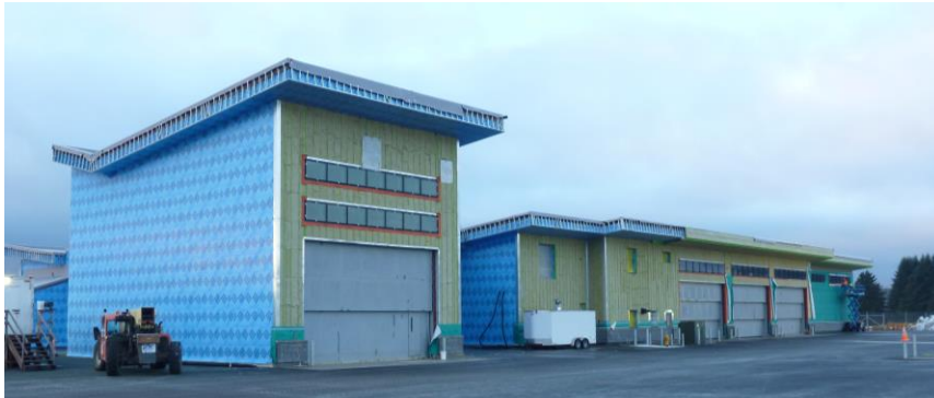
SREB exterior view from northwest corner - maintenance bay at left.
