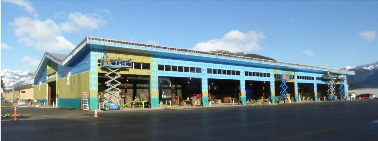
SREB exterior view from southwest corner.
