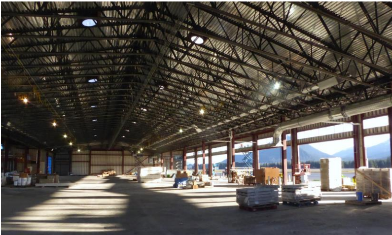
SREB interior view from west end.
