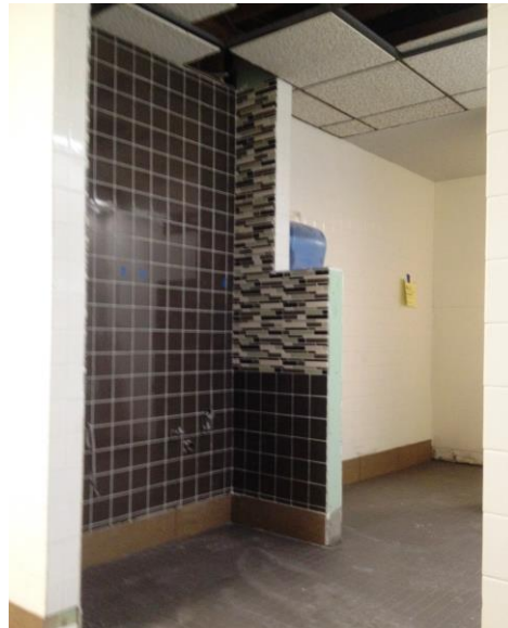
Tile installed in Men's Restroom.
