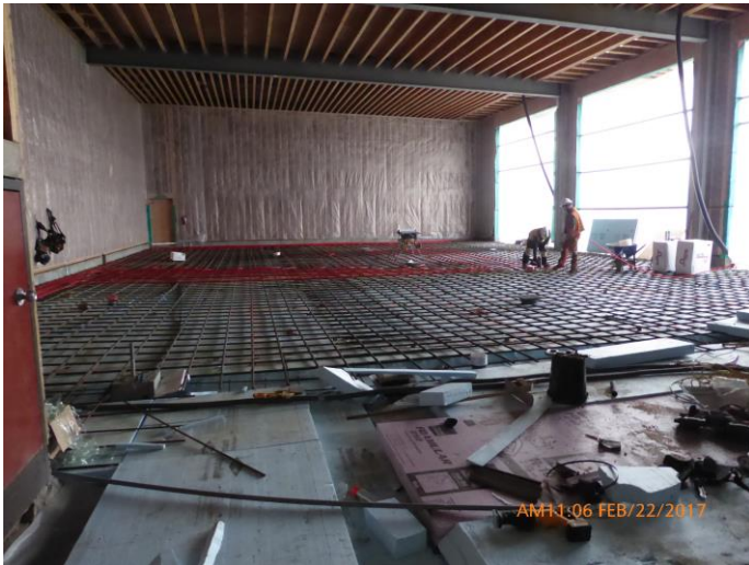
ARFF Station floor slab preparation.
