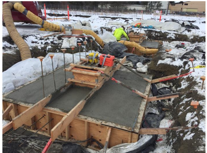
SREB concrete foundations.
