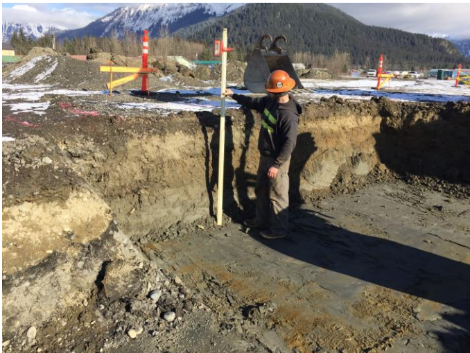
SREB excavation for foundations.
