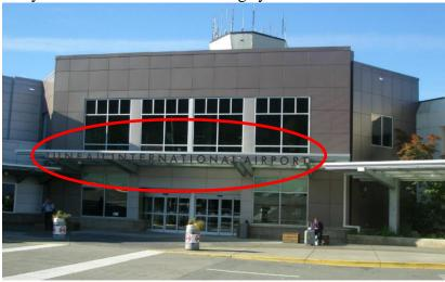
**Option B.1**: Uses 8" letters directly mounted to the siding above the entry doors. This concept will require that the siding around the entry be removed to place blocking into which the letters will be fastened.
