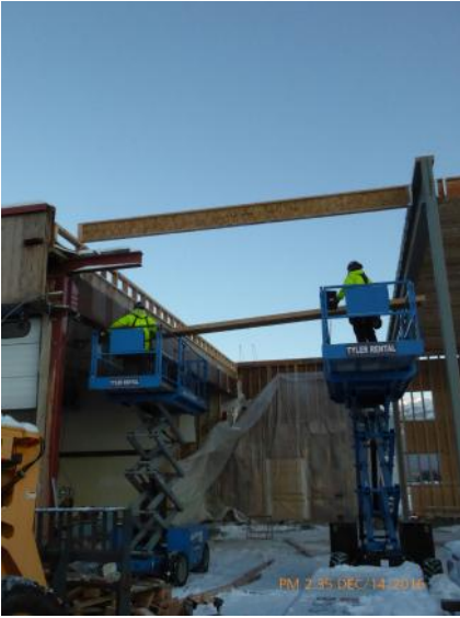
Roof joists being raised at ARFF station.
