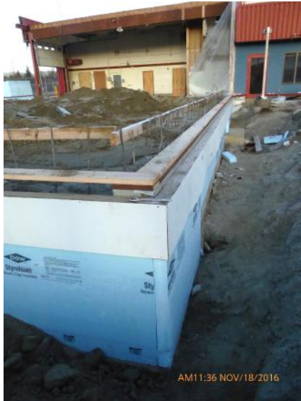
Insulated stem wall at ARFF station.
