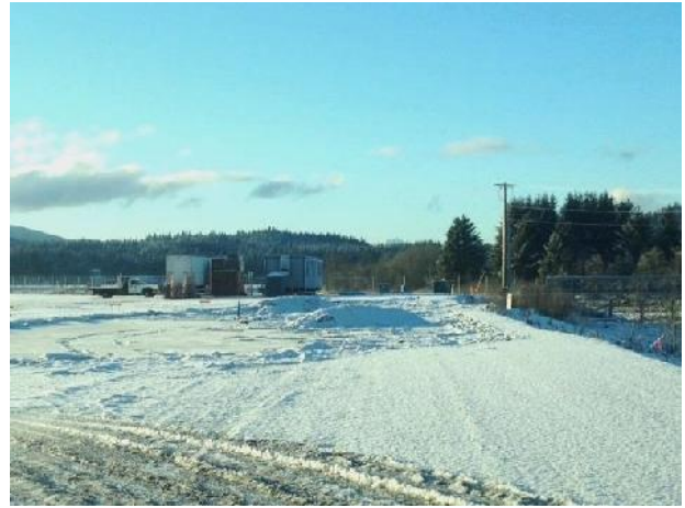
Job trailers are set at NW corner of SREB site.
