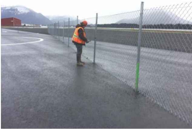
SREB construction area fencing being installed.
