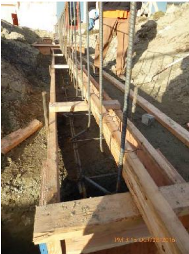
New footings being formed at station
