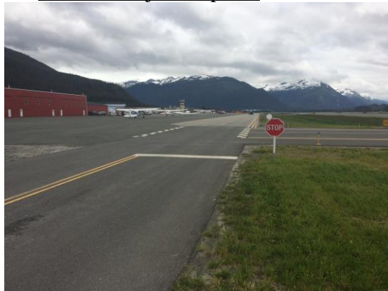
Frangible stop signs on roadways.
