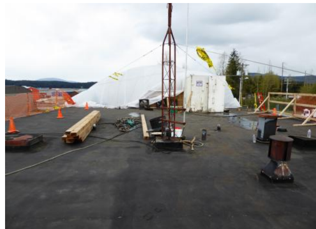
Active work area is enclosed under tent.
