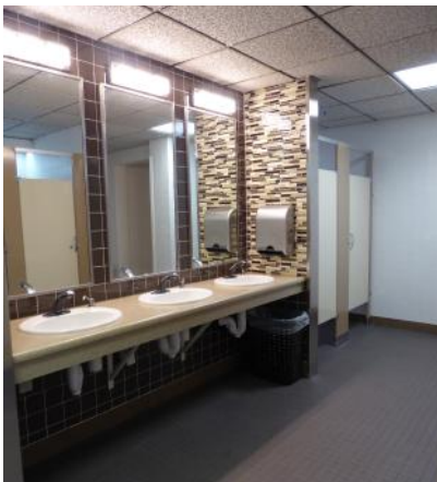
First Floor Women's Restroom complete.
