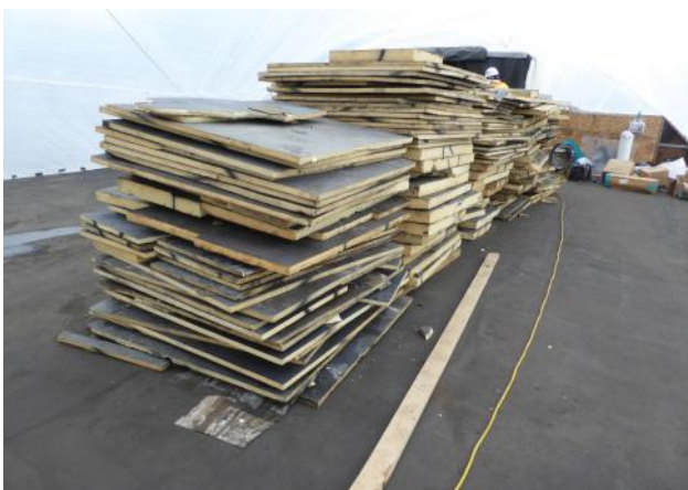
Sections of old roof are cut out and removed.
