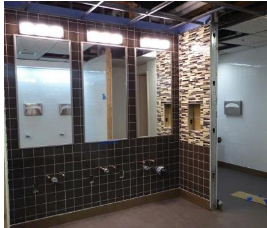
New lavatory wall is ready to receive counter top and sinks.
