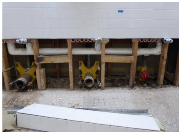
Circa 1957 toilet fixture carriers are exposed. These will be replaced.
