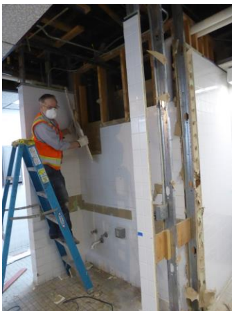
Tile demolition in progress.
