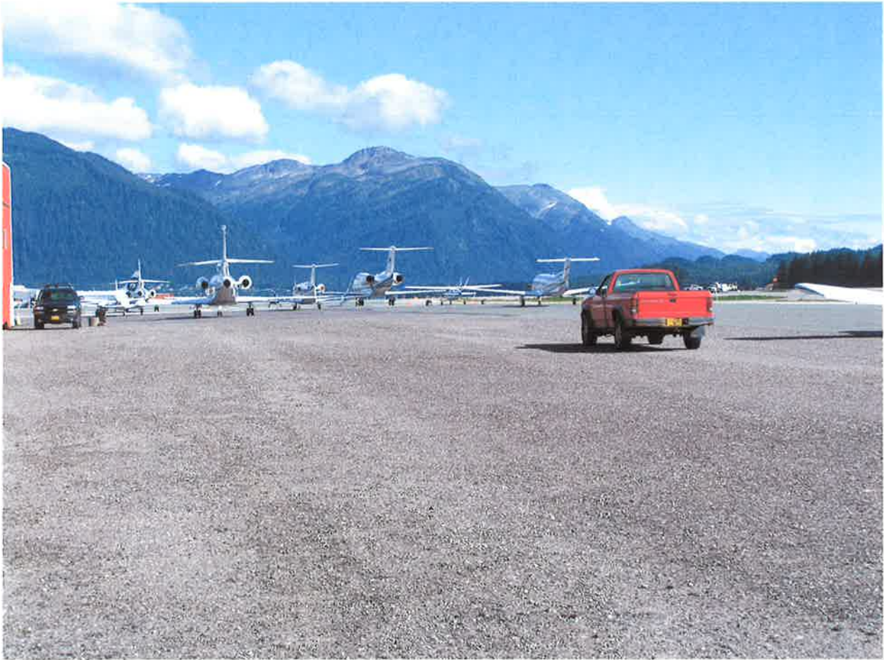
Plugged Aero Services Area
