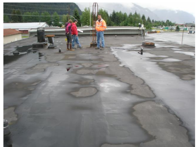
Roof conditions are noted in a June 5 review with contractor.
