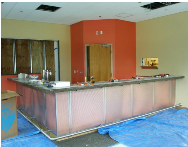
New Bar is nearly ready for final clean up and inspections.
