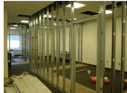
Wall framing for new offices.
