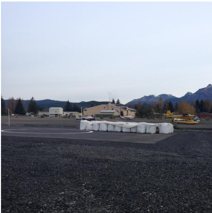
Contaminated Soil Staged on Temporary Helipads
