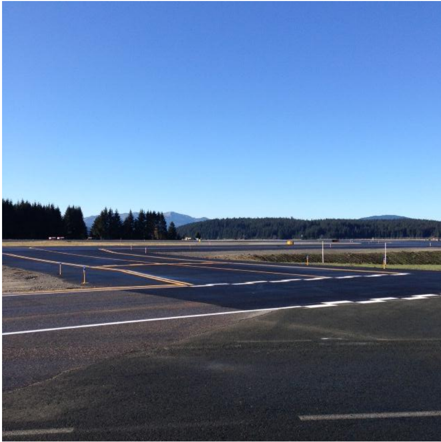
Reconstructed Taxiway B-1
