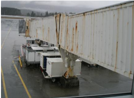
Existing Gate 5 jet bridge
