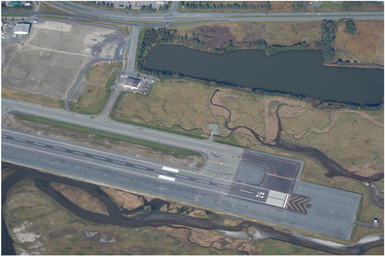
East End Runway Safety Area
