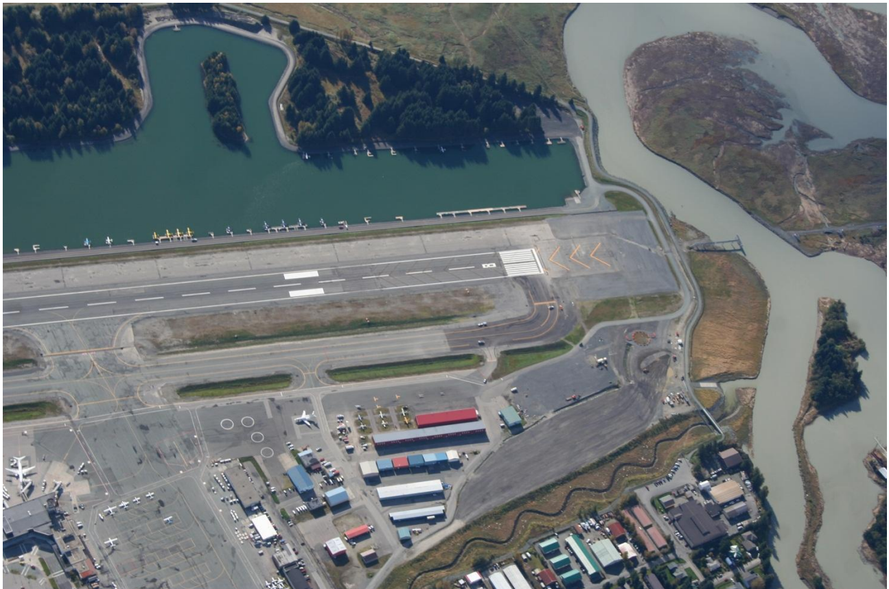
West End Runway Safety Area, Taxiway B Reconfiguration, and Northwest Development Area
