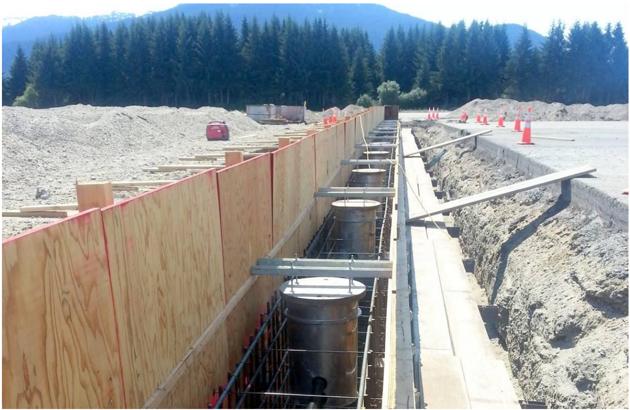
Runway 8 Threshold Installation
