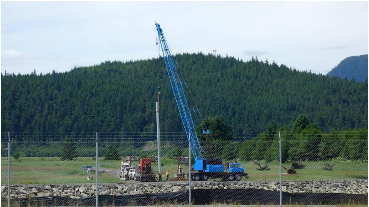
Pile Driving for the new 8 MALSR System
