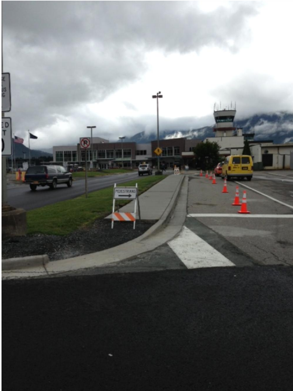
Sidewalk Installed North of Terminal (Pedestrian Ramp not yet completed)
