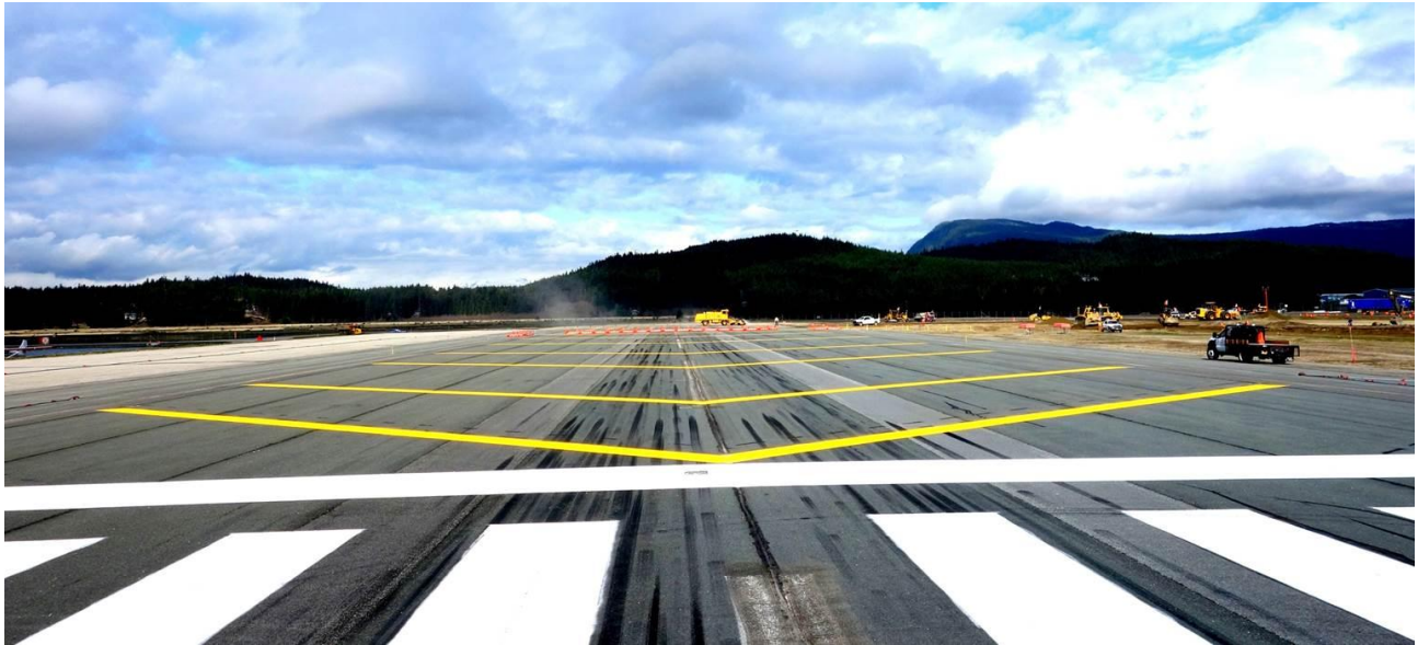
Runway 8 Relocated Threshold.
