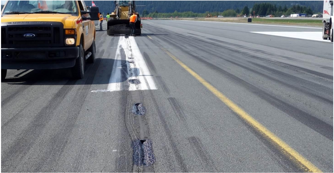
Runway Emergency Centerline Patching
