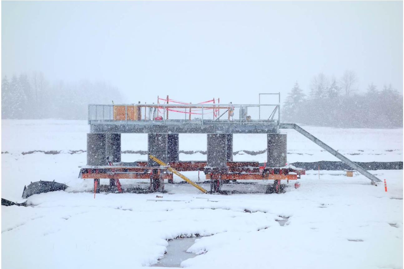
Construction of the 26 MALS platform at Station 8
