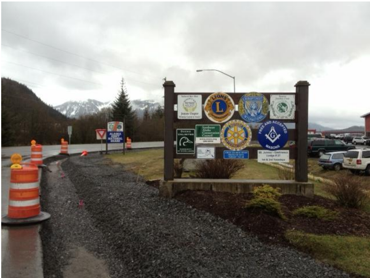
Base rock installed for curb/gutter/sidewalk on outbound Shell Simmons
