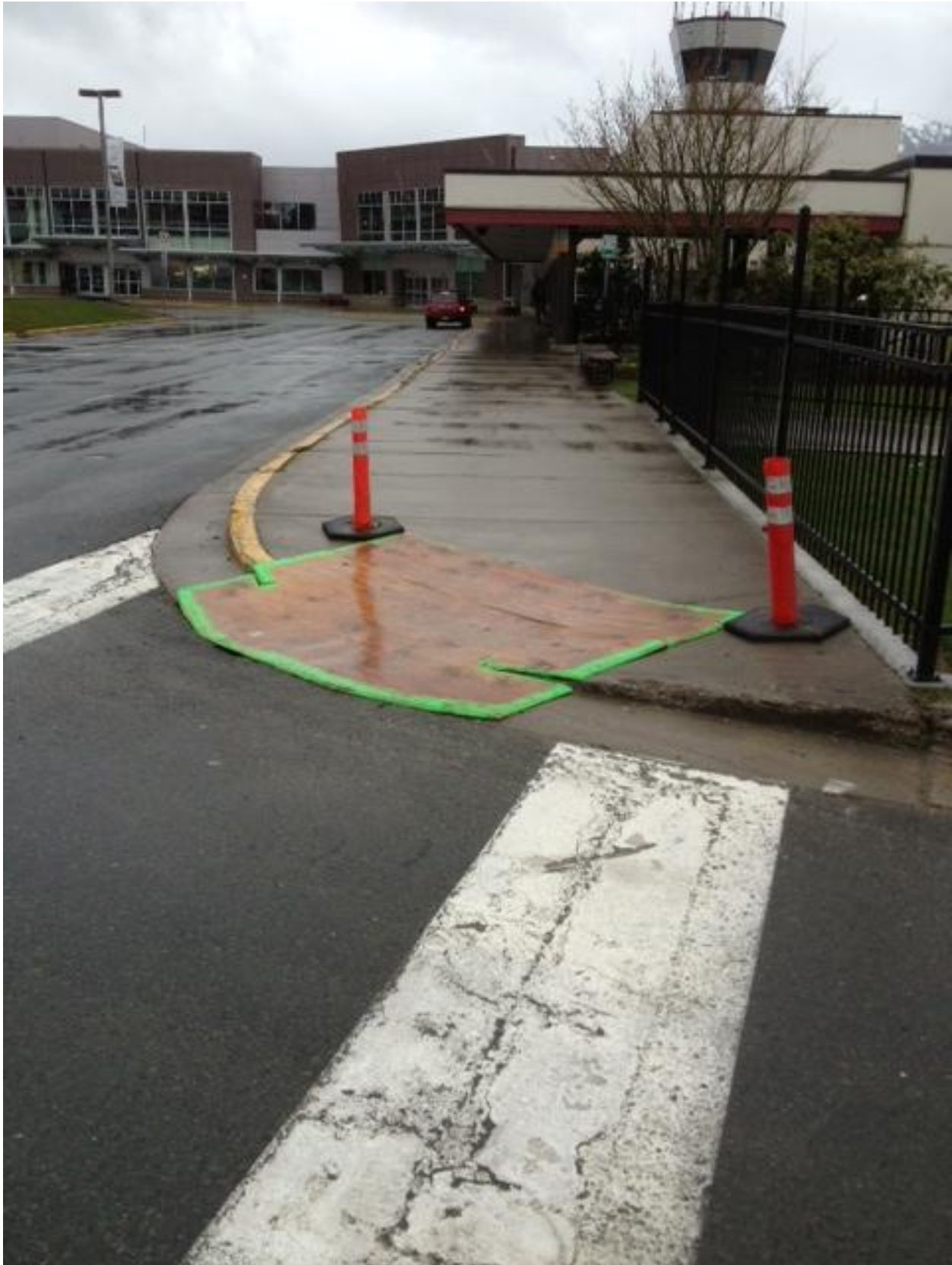
Temporary pedestrian ramp leading to the terminal.
