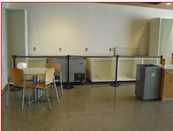
Construction underway for Departure Lounge coffee bar.
