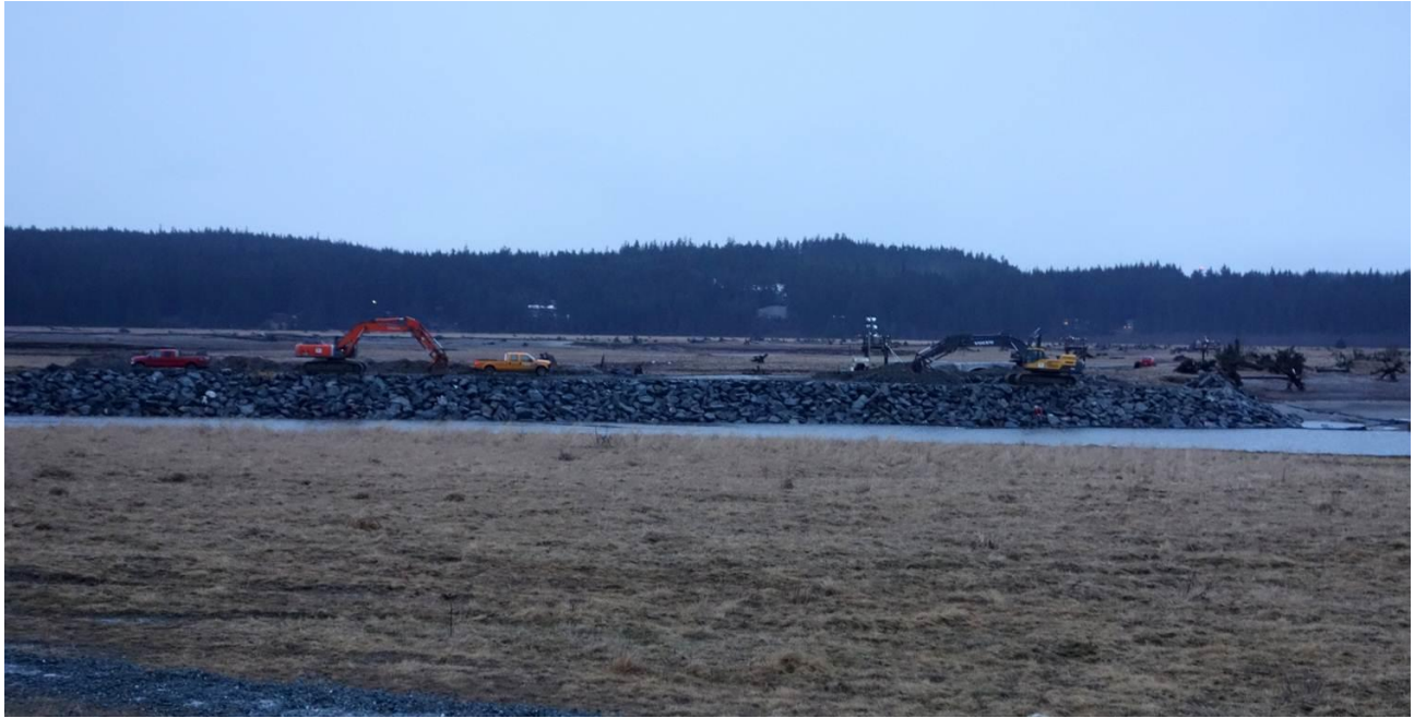
Construction work on removal of the “thumb”
