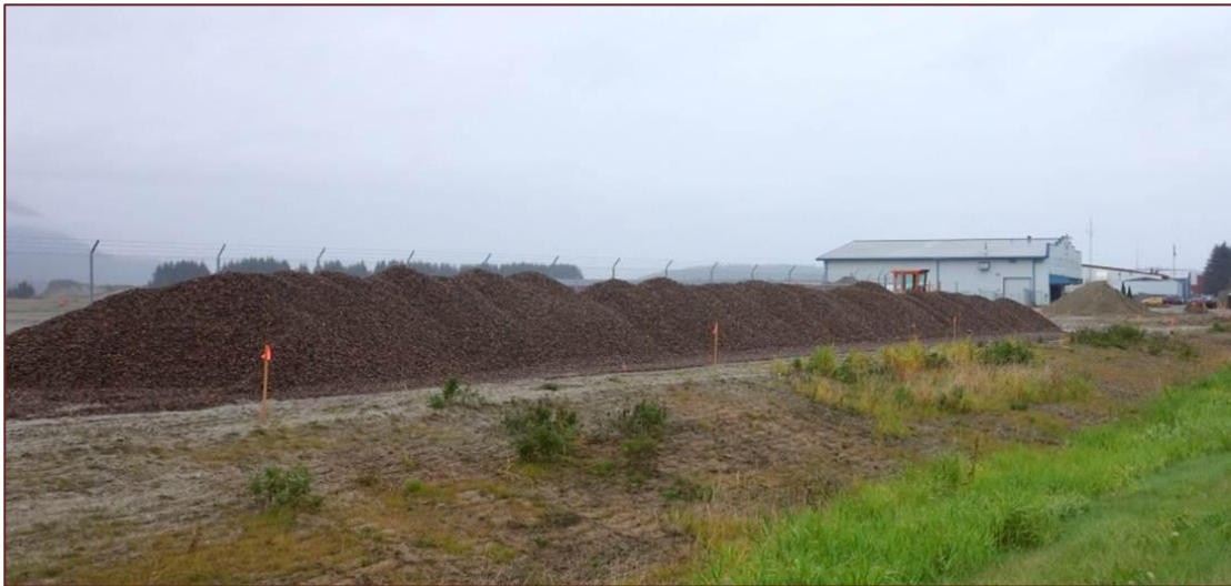
SREF roadbed material is stockpiled on the site.
