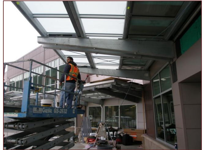
Electrician works on lights and speakers under new canopy.
