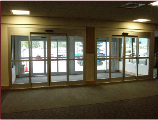
Lobby & vestibule complete, except for stone tile on center column.
