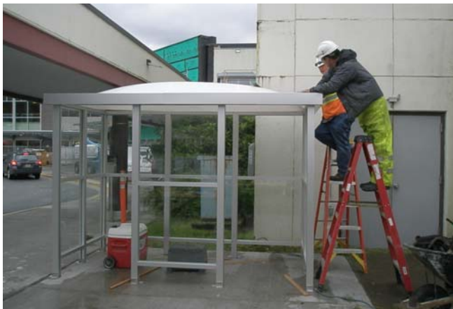
ASRC McGraw carpenters assemble the Smoking shelter
